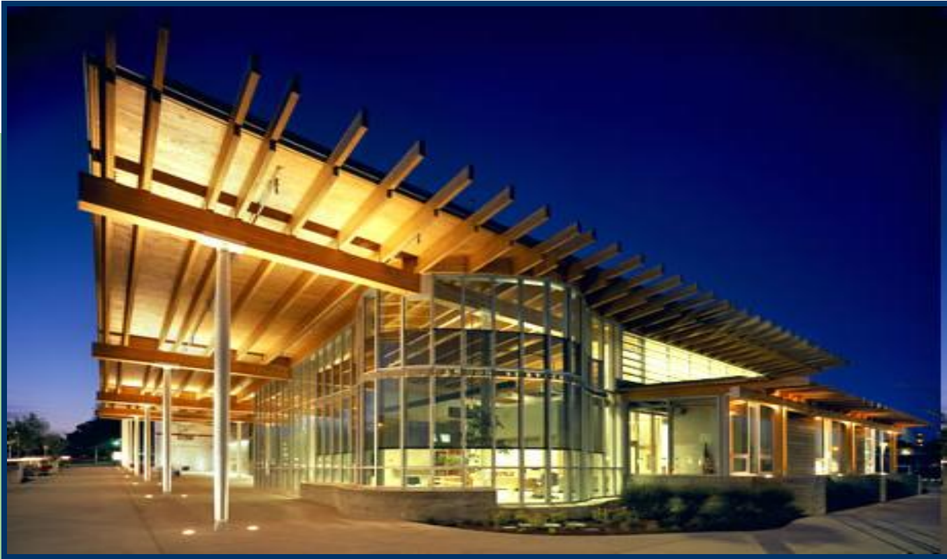
Ballard Library in Seattle. A state-of-the-art green building which makes use of a sod roof, daylighting, and translucent thin-film solar collectors. It is listed in the American Institute of Architecture's top ten green buildings.
